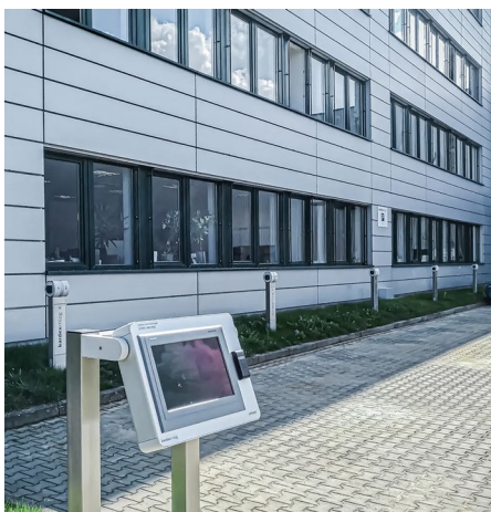
Fig. 5 Charging stations in Neuenstadt (Germany)
